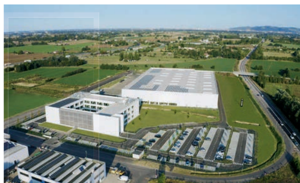
VGP Park Valsamoggia, Bologna, Macron Headquarters
